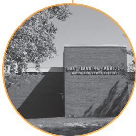
2470 Burcham Dr., is operated by the East Lansing-Meridian Water and Sewer Authority (ELMWSA).
